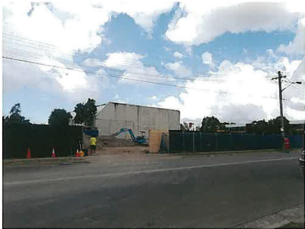
Figure 17: 1-9 Monash Road (mixed use development under construction)
